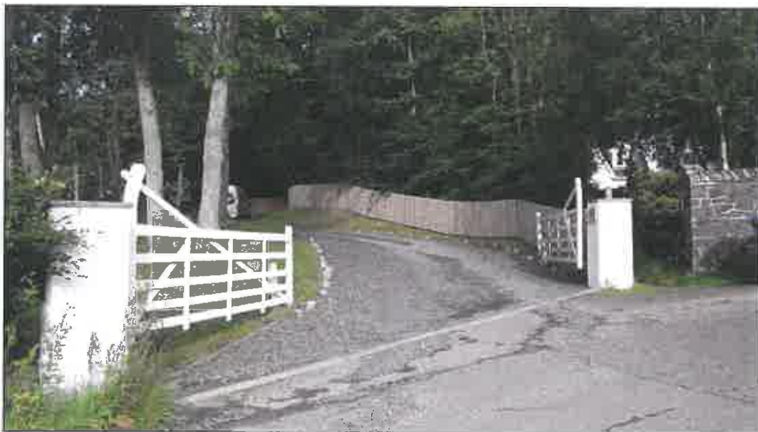
Fig 6: Access into Craigerne Coach House which will be used by the plot
